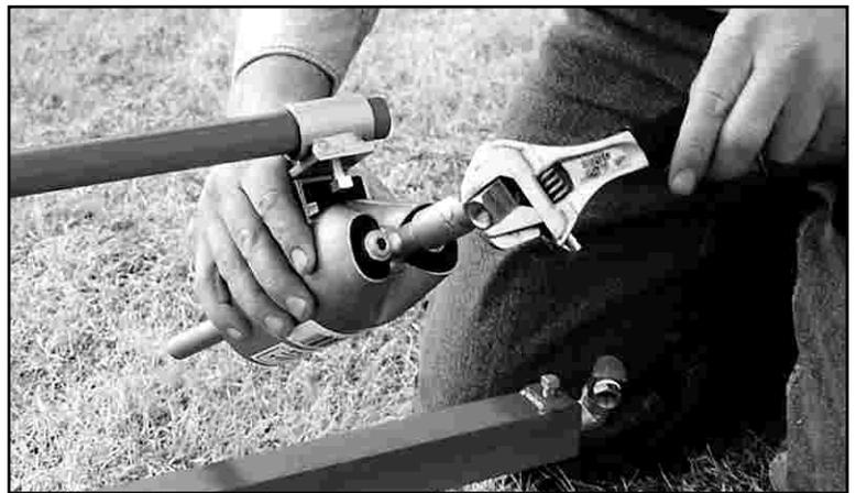
**10)** Slide 35" nipple through top hole of skid and using thread sealant tighten nipple into torch elbows. Repeat for other side.
